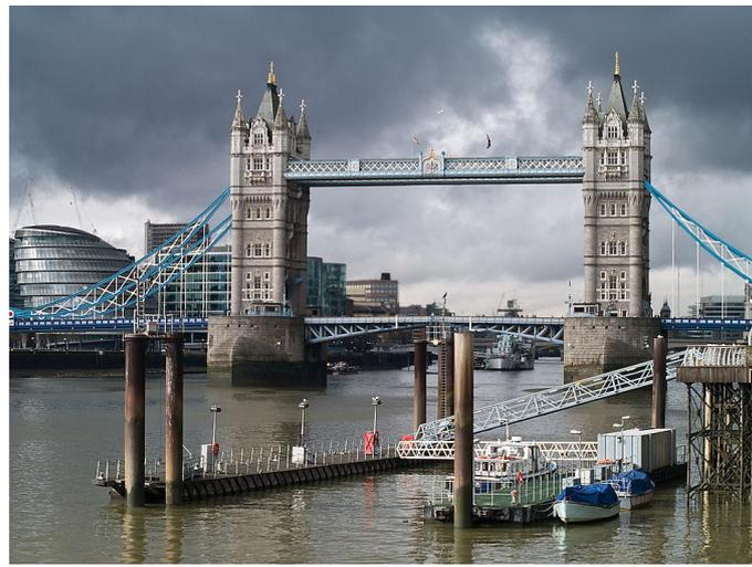
**The bridge was actually built in the late 19th century – and it’s a feat of Victorian engineering. It’s not a drawbridge, but instead features a ‘bascule’ bridge (a French word for seesaw). Both sides of the road open on a pivot, letting cargo**
